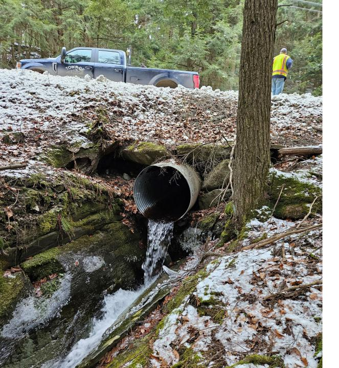
Belgo Road Culvert to be replaced with a new structure that meets current design standards and has appropriate bankfull width.
